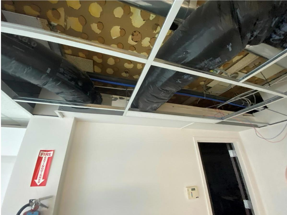
Photo No. 2: Existing 2<sup>nd</sup> Floor Dual Ceiling with Low Ductwork Conditions
